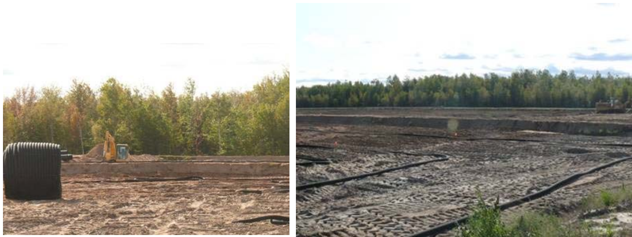
Figure 7. Installation des drains
